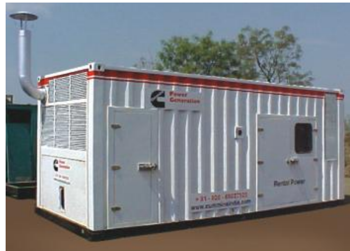
500 kVA Power Box - A recent addition to meet the plant's expansion
