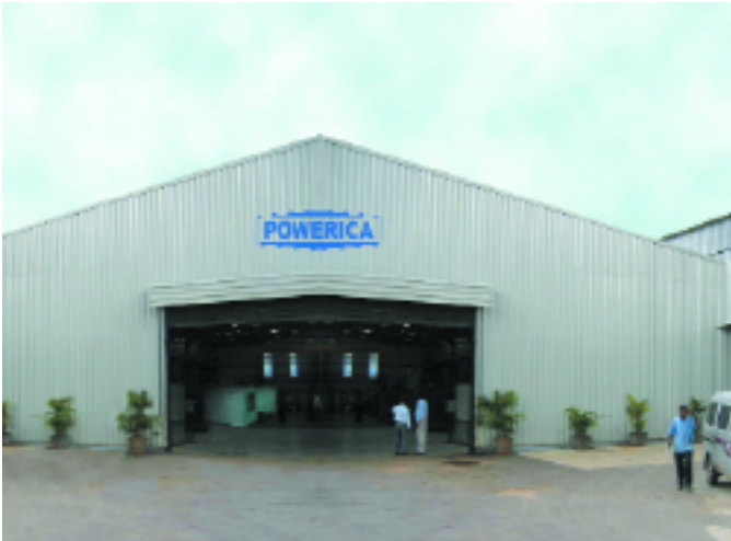
Facility at Bangalore
