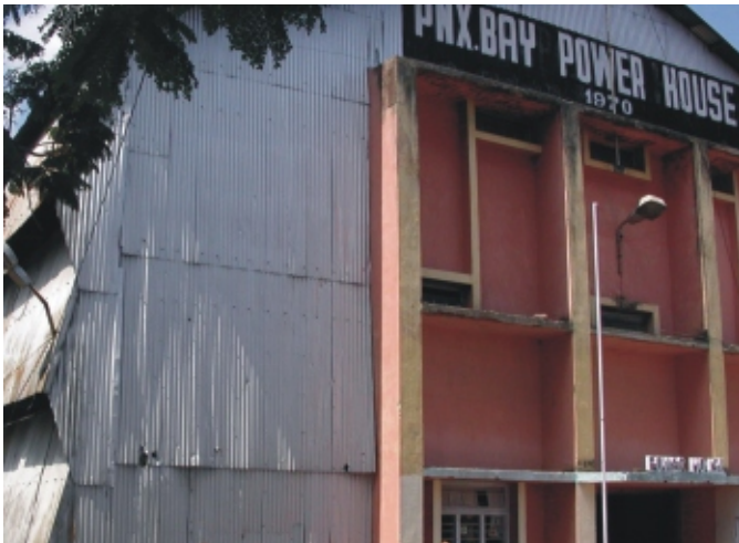
Powerhouse at Phoenix Bay
