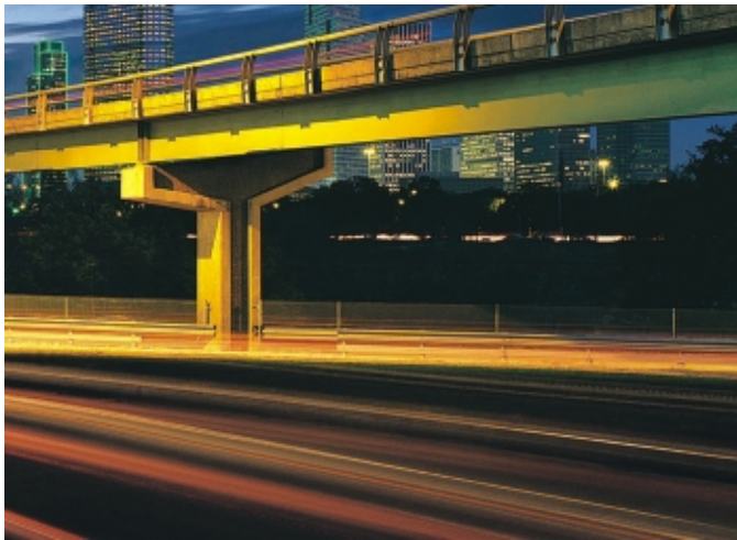
The Noida Toll Bridge, an eight lane bridge-cum-expressway project powered by Cummins gensets
