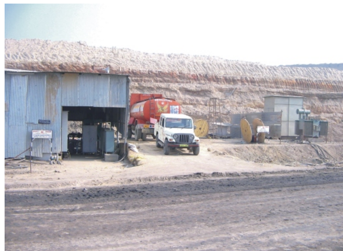
Fuel handling system with ramp to facilitate gravity flow to day tanks
